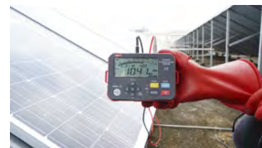
Energized device test (DC 1000V; PV)
