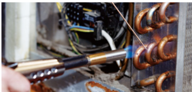
Brazing in refrigeration / air-conditioning technology
