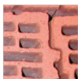
Hollow brickwork
